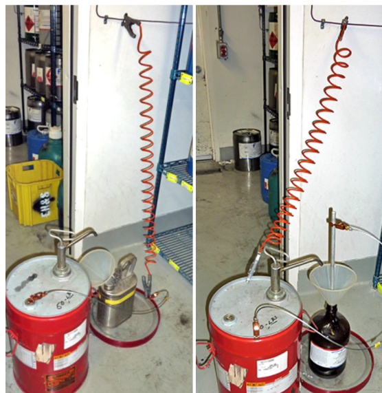
Figure 3: Shows two examples of bonding and grounding. The image on right shows dispensing into a glass container with a ground rod inserted into the funnel.
